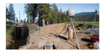
Figure 3.24: Site GASB in Alder Springs, CA. Left: Wide view showing seismic vault, which is cemented to bedrock. Right: Close-up of monument during pouring of stabilizing cement; the central support mast was embedded in the wall of the seismic vault during construction.
