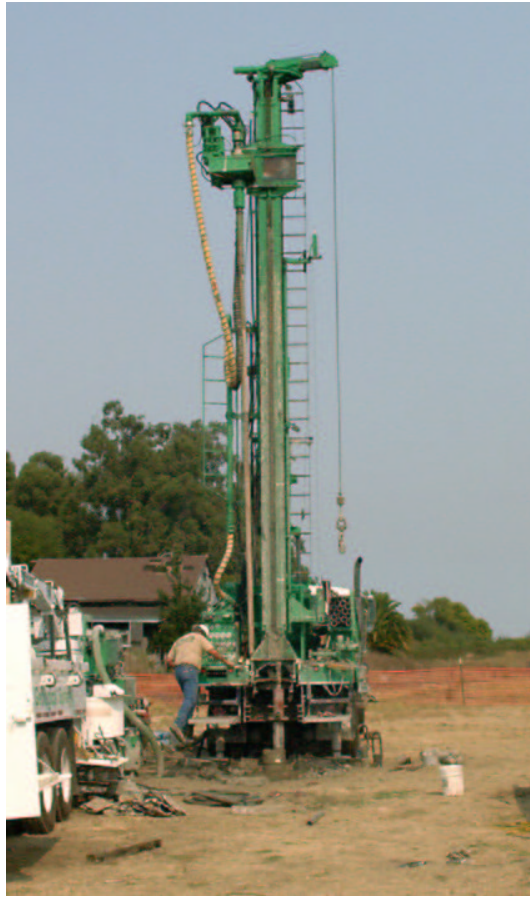
Figure 9.2: USGS Water Resources Division rig used to drill the Mini-PBO boreholes at the St. Vincents site.
