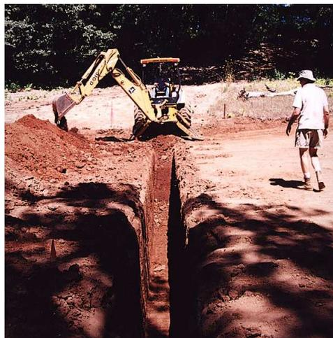
After successfully observing the interface response with the one-trench geometry (**Figures 7 and 8**), we constructed a second trench (**Figure 9**) approximately two meters from the first, in order to increase the experiment complexity. It is deeper ( $\sim 3$ m deep in the center), narrower ( $\sim 0.5$ m wide), and lacks the plastic sheeting that lines the first trench.
