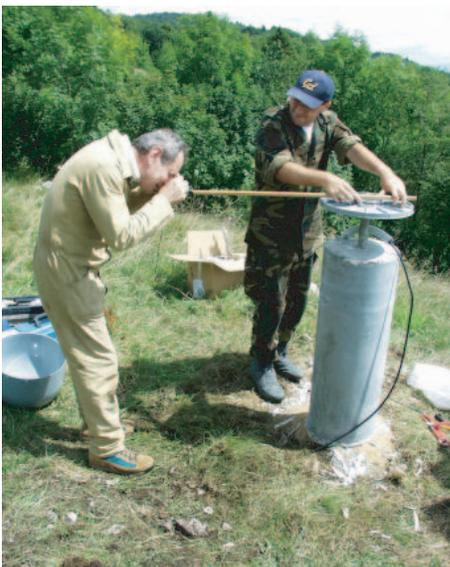
Figure 15.30: Installation of the GPS monument at MPRI. Concrete pier is tied to near surface bedrock using epoxied steel bars. A compass attached to a wooden rod is here being used to orient the antenna adapter to north.
