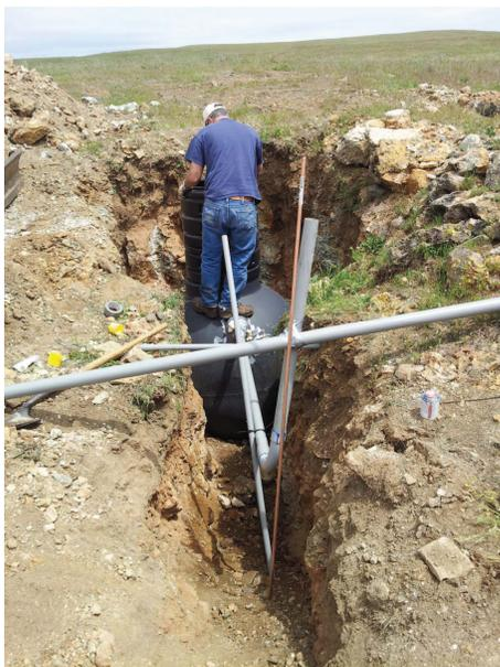
Figure 2.6: Installation of seismic vault at TremorScope station THIS.
