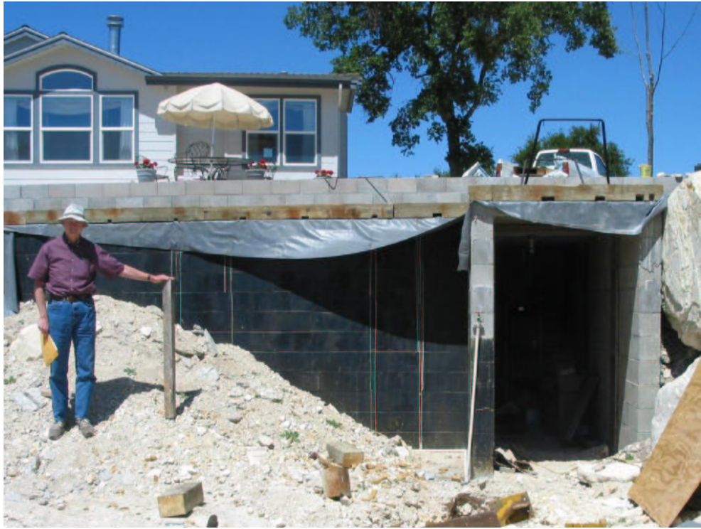
Figure R5. Proposed site of satellite telemetry dish in from of the new shop at the Ramage residence. The plan is to install the dish so that it will not be visible from the residence.
