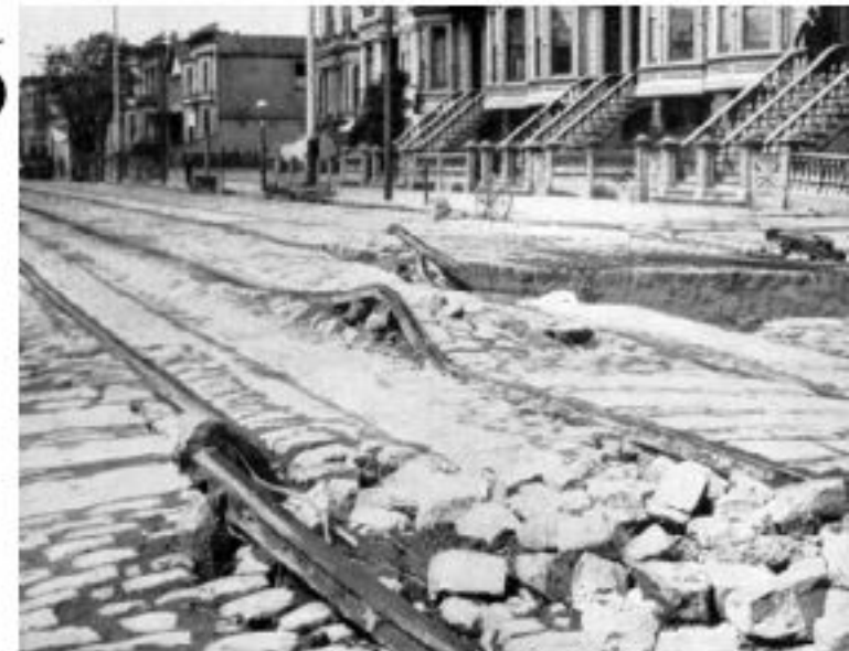
Howard Street Buckling caused to earth flow
