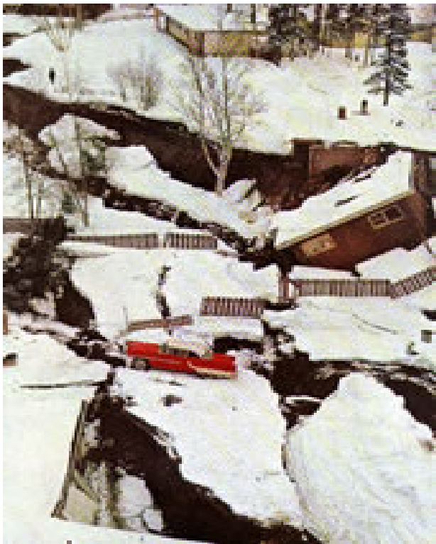
1964 Alaska (M 9.2) Ground failure
