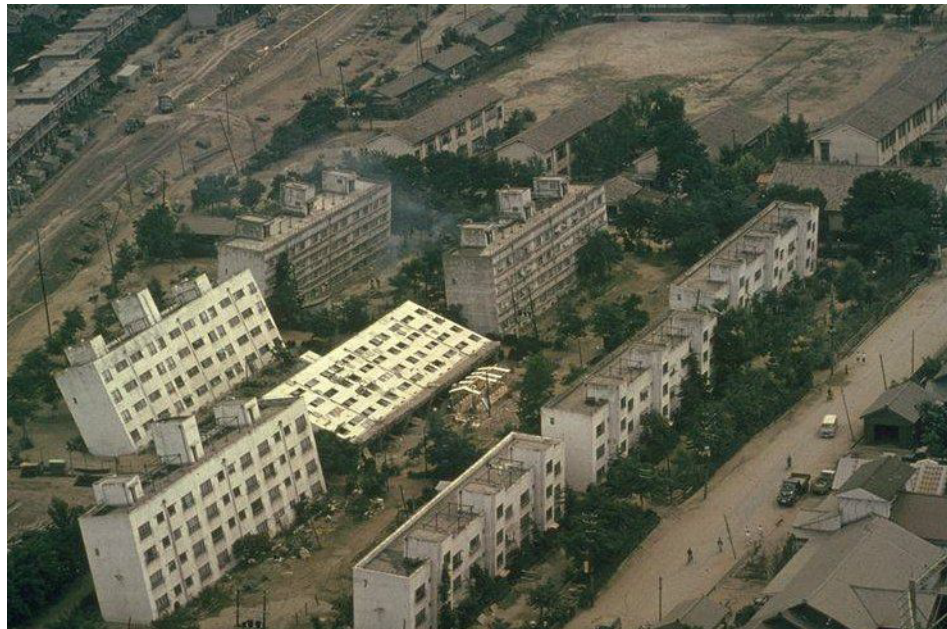
1964 Niigata (M 7.2) Liquefaction
