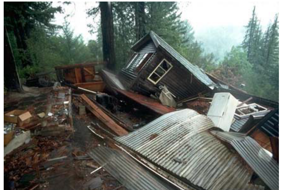
1989 Loma Prieta (M 7.9) Ground failure in Santa Cruz mountains
