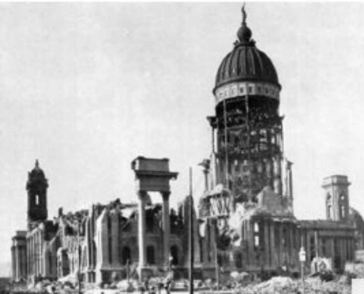
San Francisco City Hall Poor workmanship, material and design
