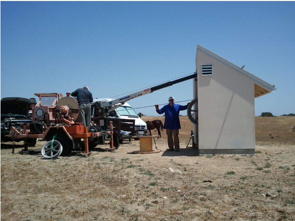
Figure 2.45.2: Installing borehole sensors at TCAS
