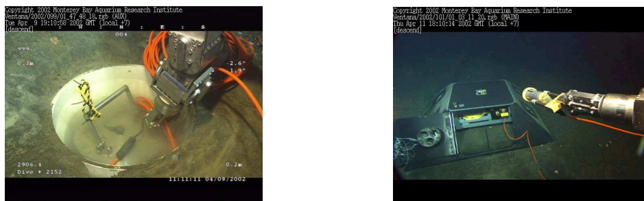
Figure 2: left: Installation of the seismometer package inside the PVC caisson. This was later completely covered by glass beads. Right: Trawl-resistant enclosure for the recording and battery packages. This snapshot was taken as the ROV Ventana was bringing the cable from the seismometer package in order to connect it onto the recording package. The first time such a remote underwater connection was attempted during the MOISE experiment, it took 2.5 hours to succeed and led to a redesign of the geometry of the instrument packages. The ROV operators are now able to do this routinely in less than 5-10mn.
