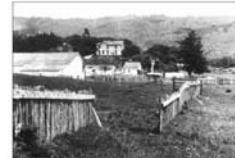
A fence built across the San Andreas fault near Bolinas, California, is offset by nearly 3 m after the great San Francisco earthquake
